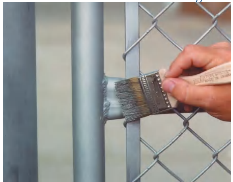
Zinc-rich Paint Application
